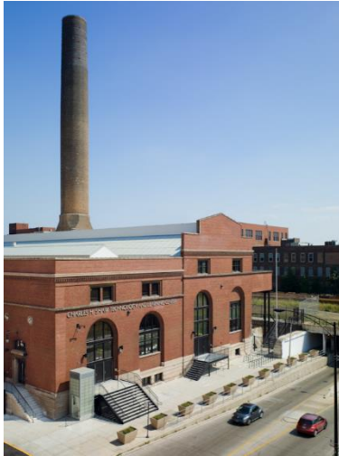
Figure 1: Homan Power House today. Image Credit: Darris Lee Harris
