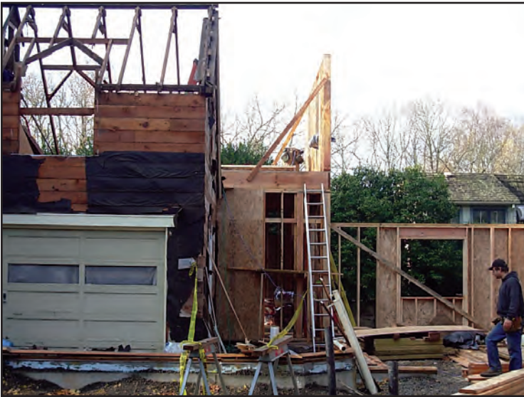
A home undergoing deconstruction. (Photo courtesy of Rebuilding Exchange.)
