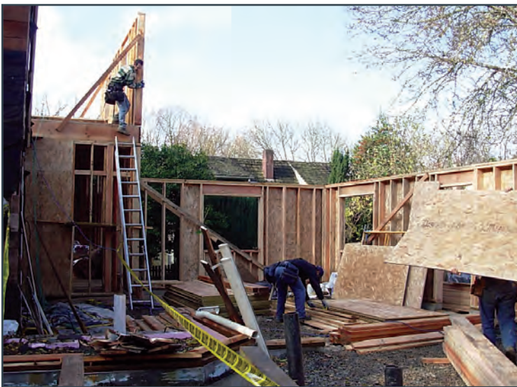
Deconstruction underway. (Photo courtesy of Rebuilding Exchange.)
