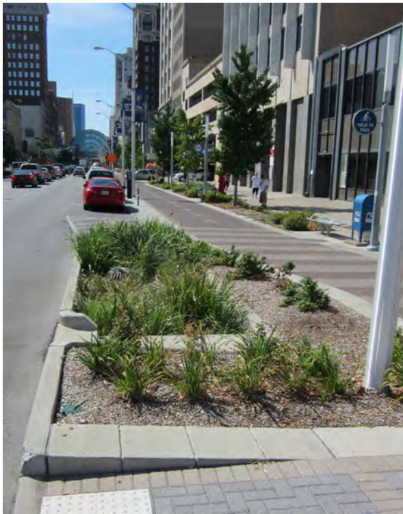
STORMWATER PLANTER INSTALLATION 5
