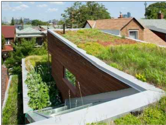
EXTENSIVE GREEN ROOF IN RESIDENTIAL INSTALLATION 1
