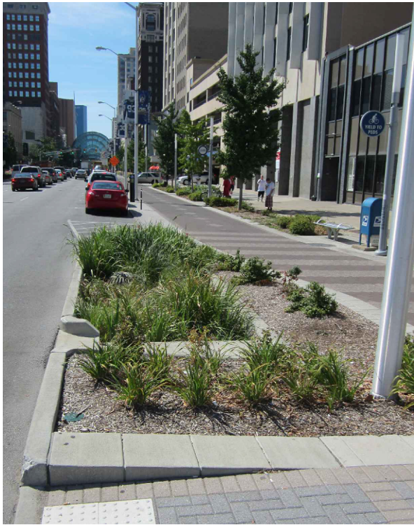
STORMWATER PLANTER INSTALLATION 5
