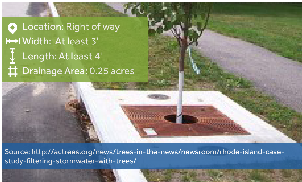
Figure 8: Box tree filter in suburban setting
