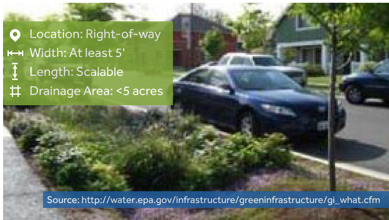
Figure 5: Bioswale in a suburban setting
