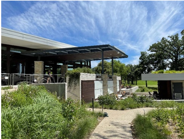
Green/Blue Roof: The Preserve at Oak Meadows in Addison, IL. Stormwater falling on the roof of the restroom building is temporarily stored and later released to roof drains or evapotranspired through the vegetation. Photo credit: FPDDC.
