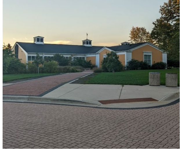
Permeable Paving: St. James Farm in Warrenville, IL. Permeable interlocking pavers allow stormwater to pass through the surface of the pavement instead of running off into the sewer or adjacent landscape. Photo credit: Kevin Dick.
