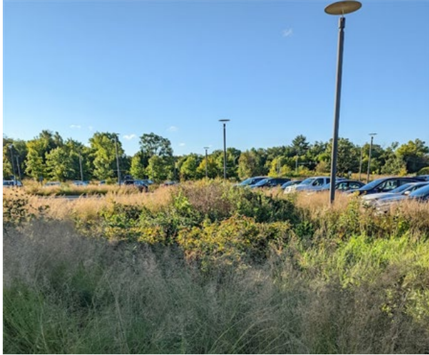
Bioretention: FPDDC Headquarters in Wheaton, IL. Runoff from the parking lot and surrounding areas is directed to bioretention islands with native plantings to filter runoff and promote infiltration. Photo credit: Kevin Dick.
