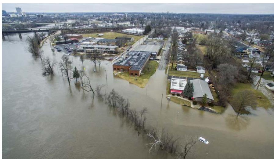
Figure 2: 2018 Flooding along Northside Boulevard in South Bend – Robert Franklin, South Bend Tribune
