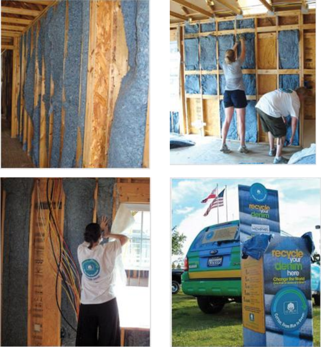
Figure 4: Using recycled denim as insulation. Source: 10.
